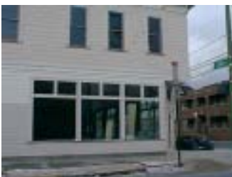
Redevelopment of the Michigan Market.
