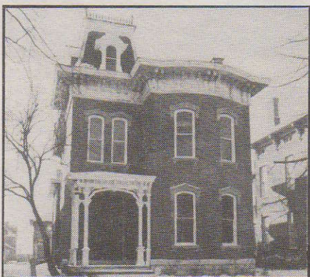
Phenomenal "in progress renovation", tower, walnut woodwork, 190's
