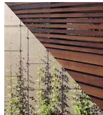
⑥ WOOD SLAT AND CABLE TRELLIS
