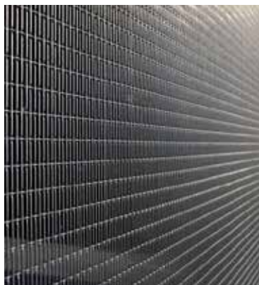
③ METAL MESH PANELS @ GARAGE
