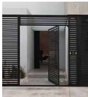
④ METAL SLAT FENCE @ COMMON SPACE ENTRY
