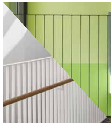
⑥ WHITE/GREEN METAL GUARDRAIL @ ELEVATED WALKWAYS & STAIRS
