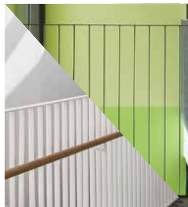
③ WHITE/GREEN METAL GUARDRAIL @ ELEVATED WALKWAYS & STAIRS
