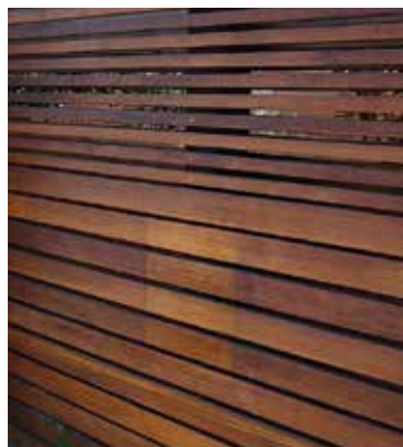
② WOOD SLAT RAIL @ PORCHES & DECKS
